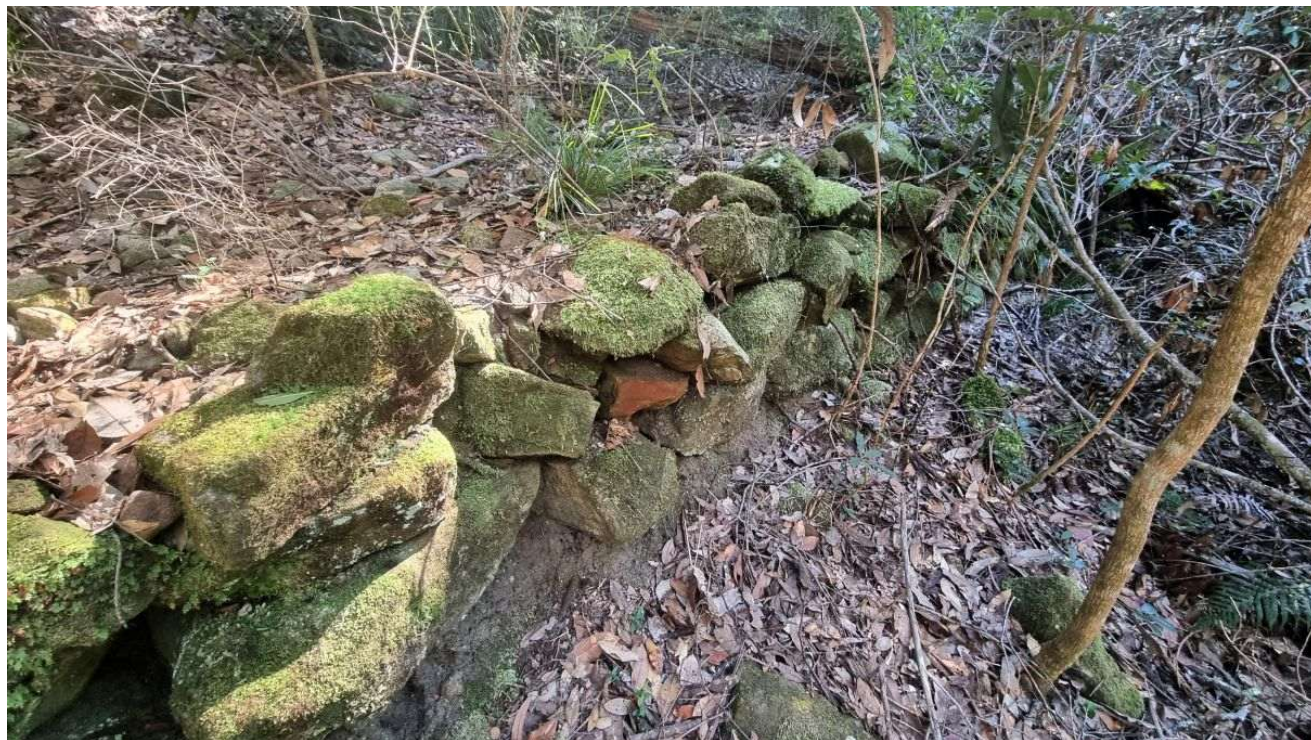
Old stone retaining wall. Photo: Yuri Bolotin.
